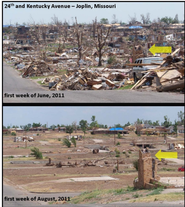
The impact of EDR on a Joplin intersection (Source: FEMA)
