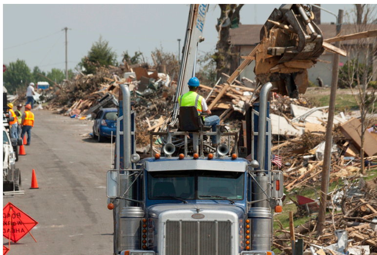
Crews remove debris in Joplin (Source: FEMA)
